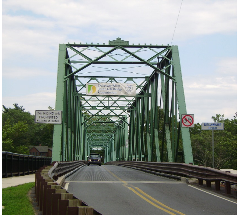
Figure 2.17 - Delaware River Bridge
