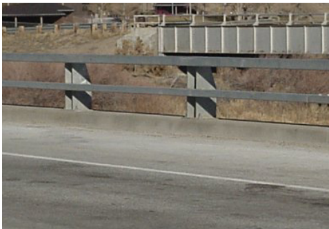
Figure 4.37 - Wyoming 2-Tube Steel Railing has a test rating of TL-4 suitable for 8000kg single unit trucks with an impact speed of 50mph.
