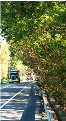
Figure 4.36 - Steel-backed wood guardrail is installed along the Delaware River Scenic Drive and should be continued into Lower Mount Bethel Township
