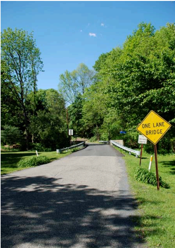
Figure 2.6 - Little Creek Road
