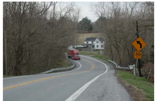
Figure 4.30 - Thicker edge line used to improve driver visibility of curve at low cost (Marland Historic National Road)
