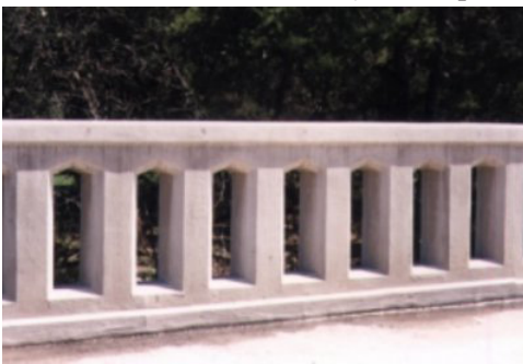
Figure 4.38 - Texas Type T411 Aesthetic Rail has a test rating of TL-2 for cars and 2000kg pickup trucks with an impact speed of 45mph. Various versions of this can be utilized to replicate some of the historic concrete bridges over Little Creek.
