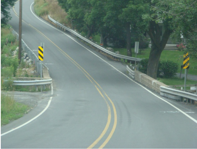
Figure 3.4 - The SR 611 Bridge over Oughoughton Creek is being rebuilt as a design build project (2011)
