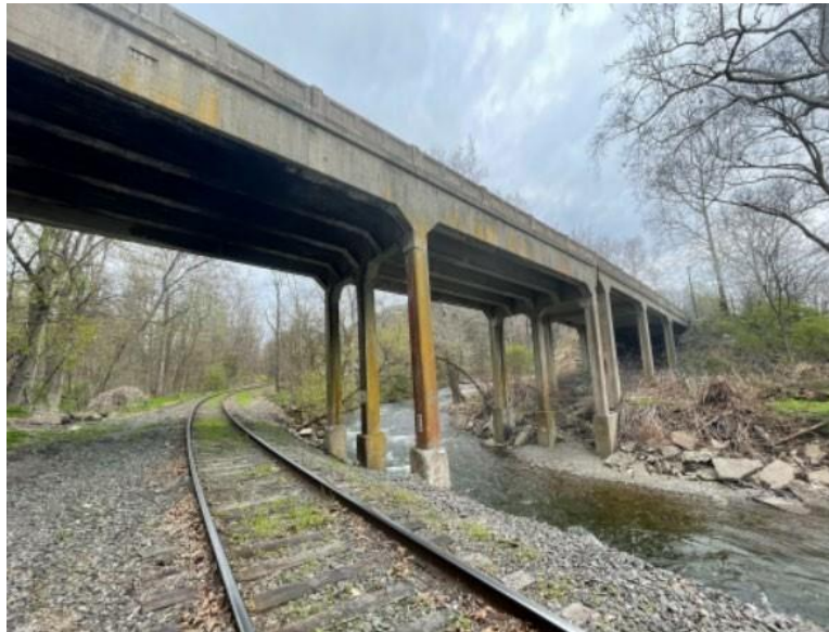
Bridge View from Pier
