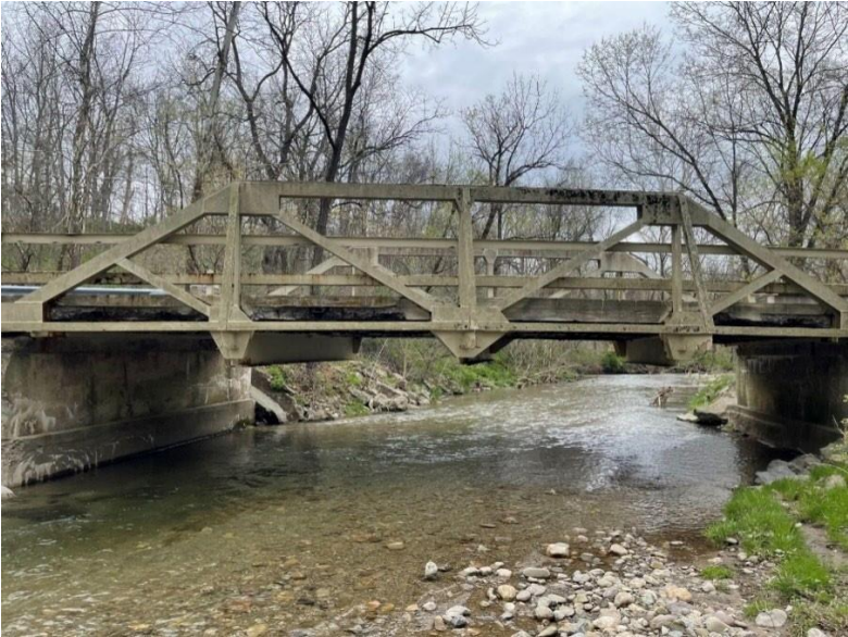
Northampton County Bridge #31
