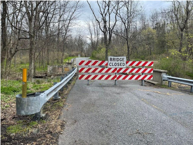
Northampton County Bridge #31
