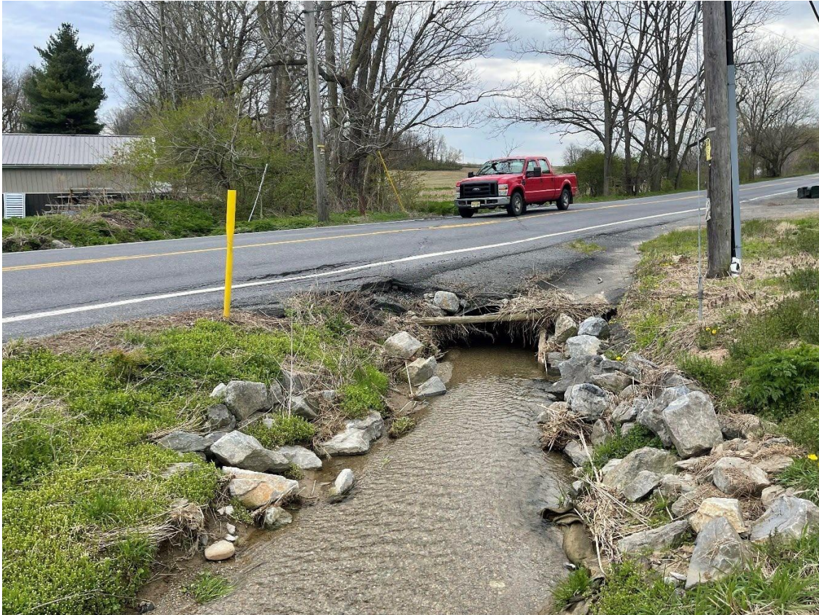
Culvert Beneath Martins-Belvidere Highway
