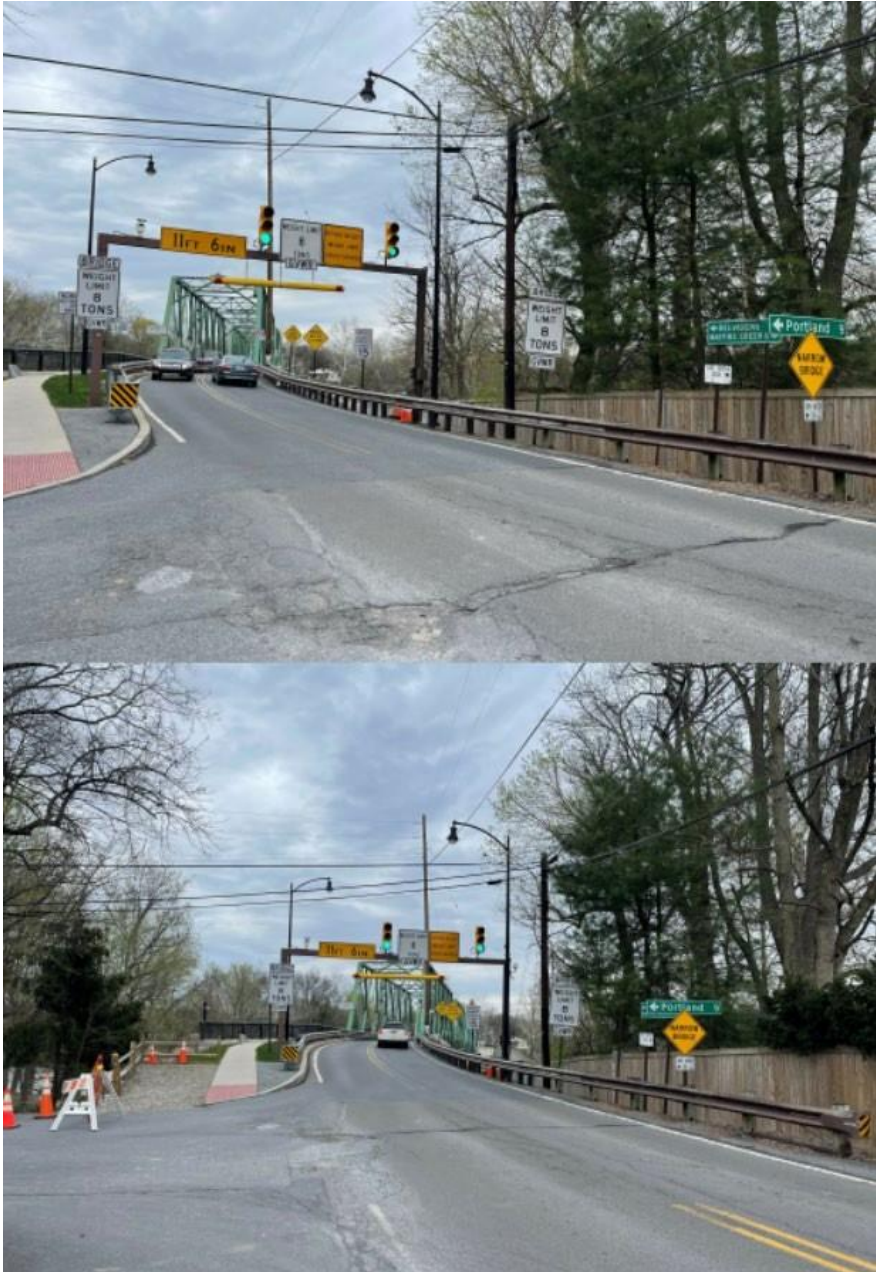
Water Street Bridge
