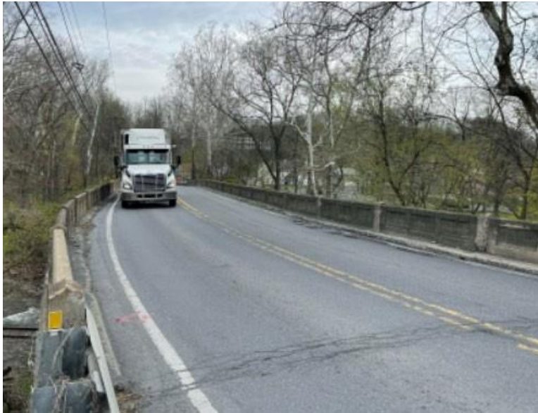
Bridge View from Deck
